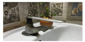
4. Using original screws and washer of tap head cover and additional washers, aluminium strip is attached firmly.
