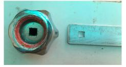
3. Tap head cover is removed. An aperture matching the tap head cover is created on the cut aluminium strip.
